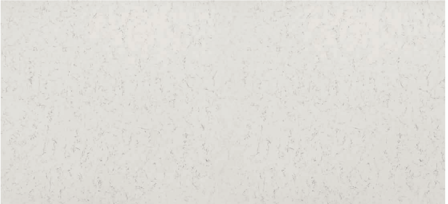
Full Slab View
