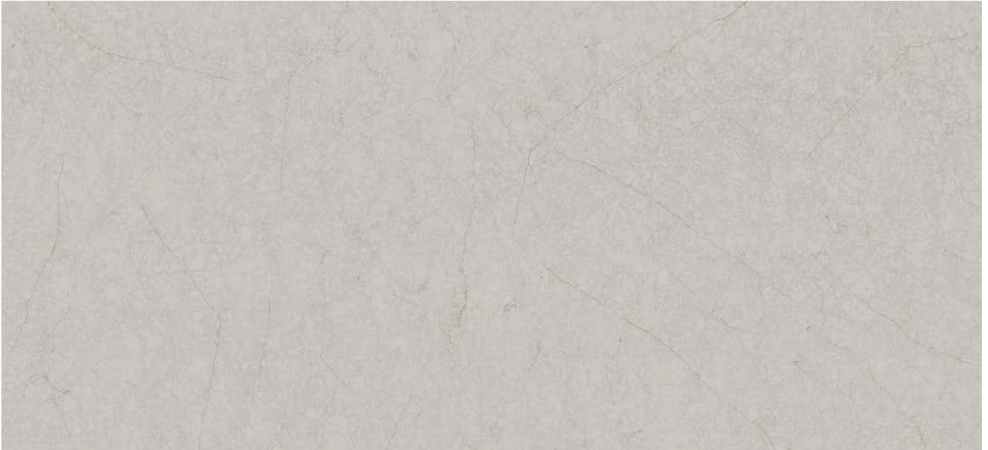
Full Slab View
