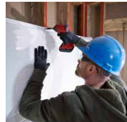
Panels fasten directly to the stud walls without adhesive
